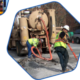
Micro Trench Installations
